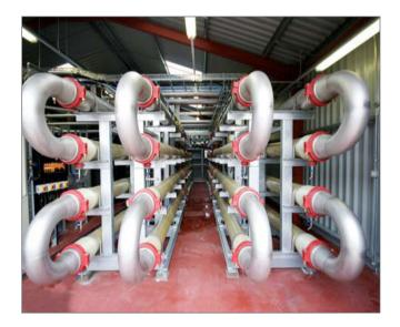
Figure 1: AMBR<sup>™</sup> UF Membrane Bank
